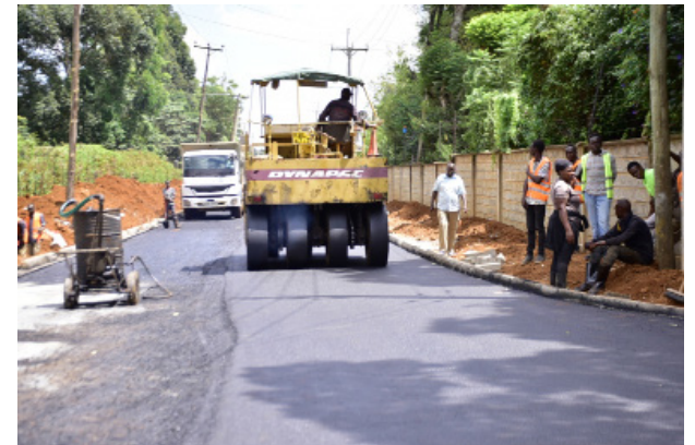
The ongoing tarmacking works of 3 Kilometres of roads in Race Course Ward, Kesses Sub County.
