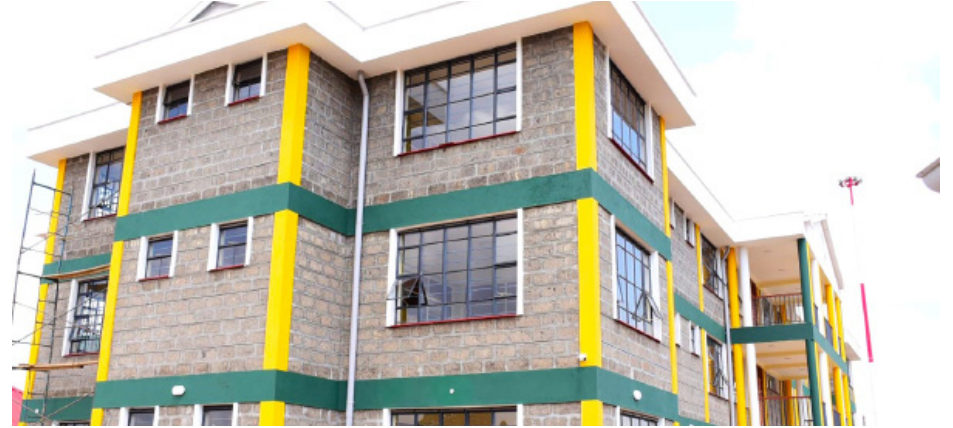
Side View of Turbo Sub-County Office.
